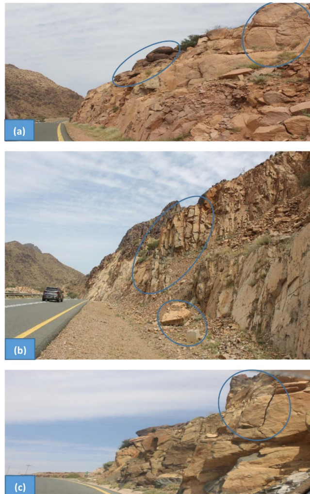
Figure 7. The internal structures that are linked to rocks and have a role in causing rock sliding. (a) Fragmented granitic blocks in the process of undergoing exfoliation and sliding. (b) Parallel and perpendicular joints are planes of weakness that can allow water to infiltrate and assist sliding. (c) A fractured granitic block located beside the road.
