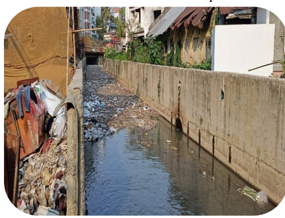
Photo-4 A congested drain in Sholoshohor
