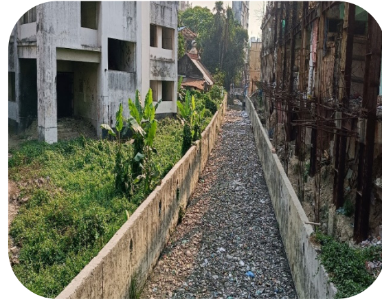
Photo-2 Water stuck due to plastic
