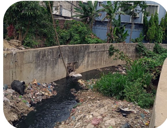
Photo-6 congestion due to siltation
