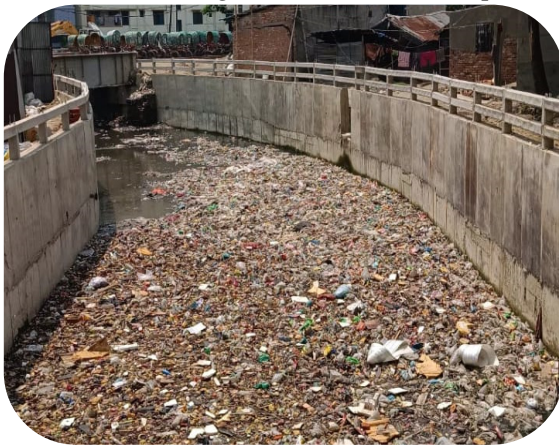
Photo-5 Water stuck due to polythene waste
