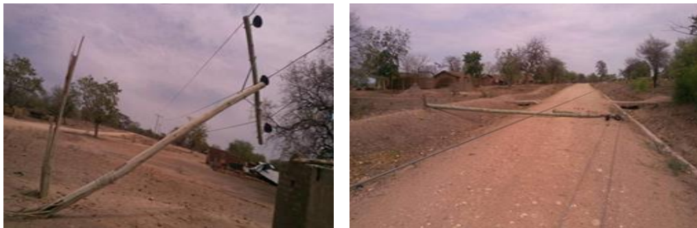
Plate 2: Electric Poles Damaged by Strong Winds in T/A Lundu
