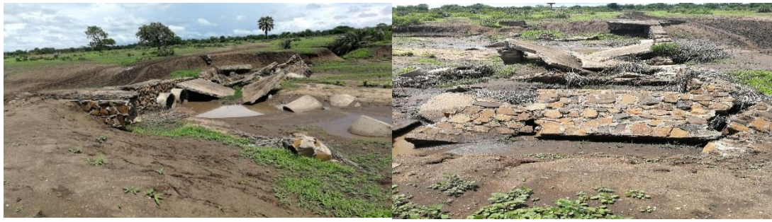
Plate 1: A Bridge Damaged by Floods at Chindoko Villagw, T/A Ngabu.
