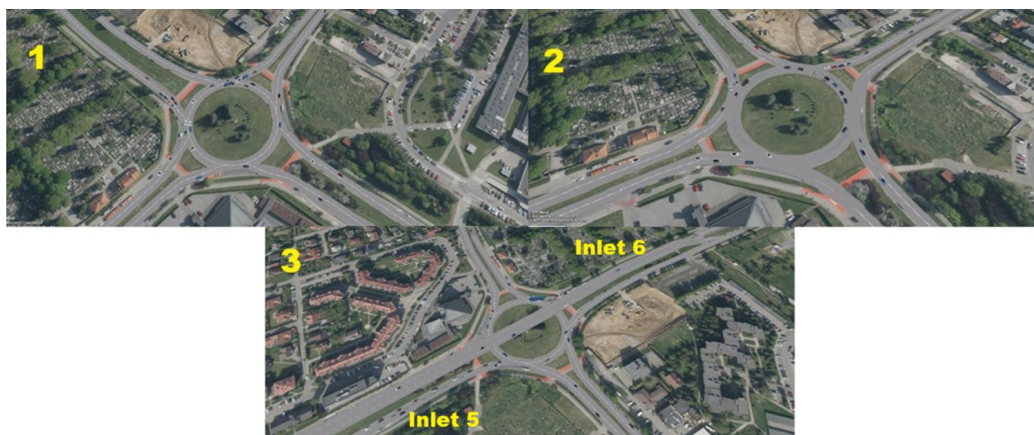
Figure 3. View of the simulated model under investigation: 1. Conventional roundabout 2. Turbo roundabout 3. Flyover-based grade-separated junction.
