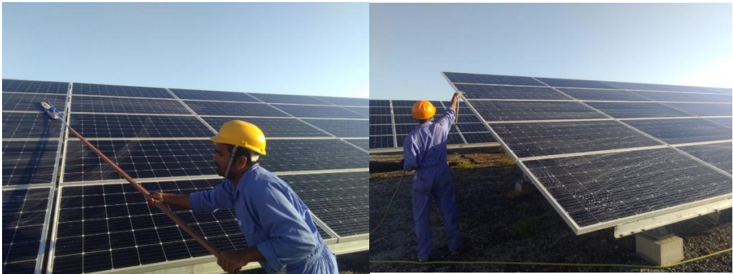
Figure 4. Manual cleaning of solar panels.
