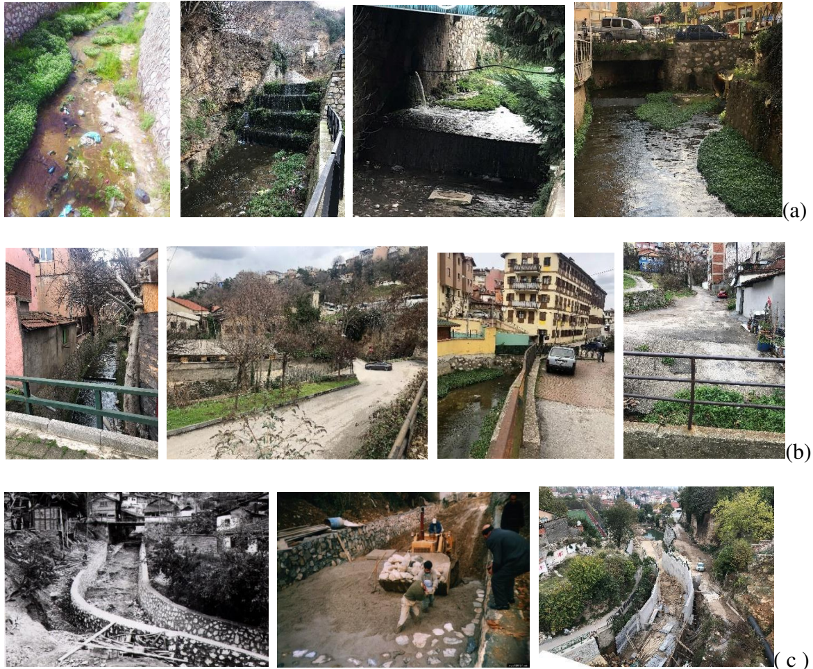
Figure 7. (a) Solid waste and water pollution within the Cilimboz Stream bed, (b) Covering the stream bed with asphalt for vehicle transportation, (c) Ground covering within the streambed with reinforced concrete and stone masonry (sources of historic photographs: archives of the State Hydraulic Works (DSİ), Bursa City Museum, and the currently photographed by the Author, 2022).
