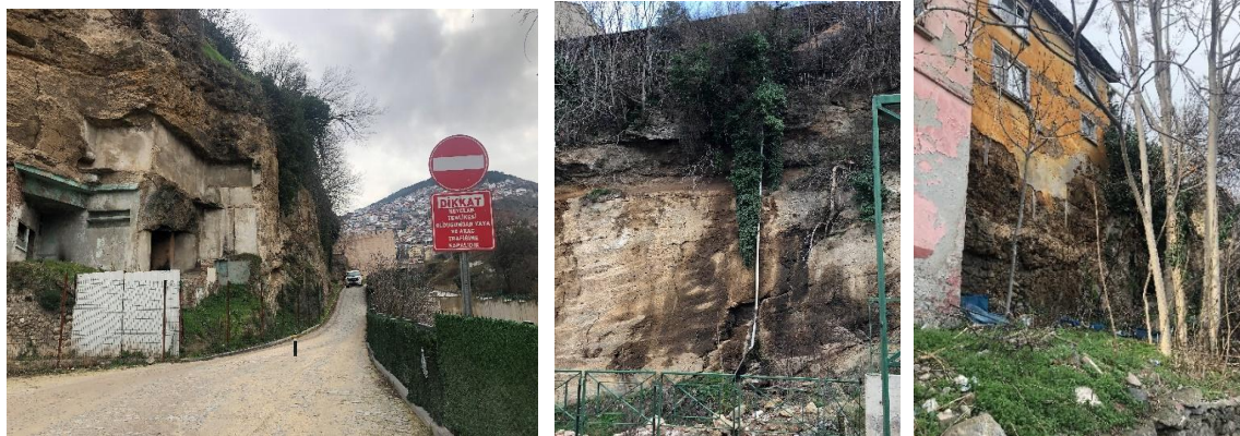
Figure 10. Facade deterioration on historic dwellings and structural cracks on the travertine cliffs, both caused by construction on the slopes of the Citadel walls (the Author, 2022).
