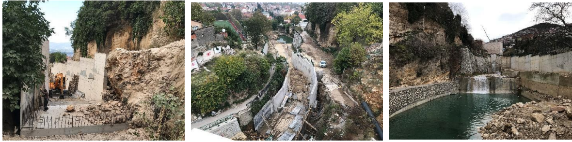
Figure 14. The process of rehabilitation; concrete covering the bottom of the Cilimboz Creek (source: the archive of DSI (the State Hydraulic Works)).
