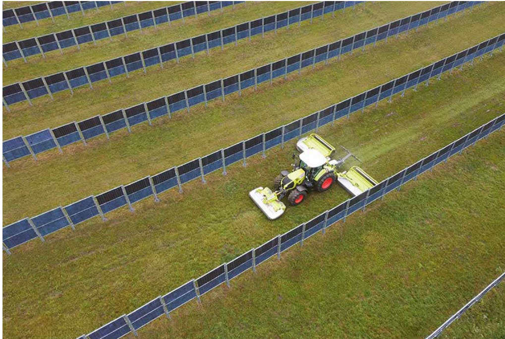
Figure 9. Reference project of the Donaueschingen-Aasen solar park [36].
