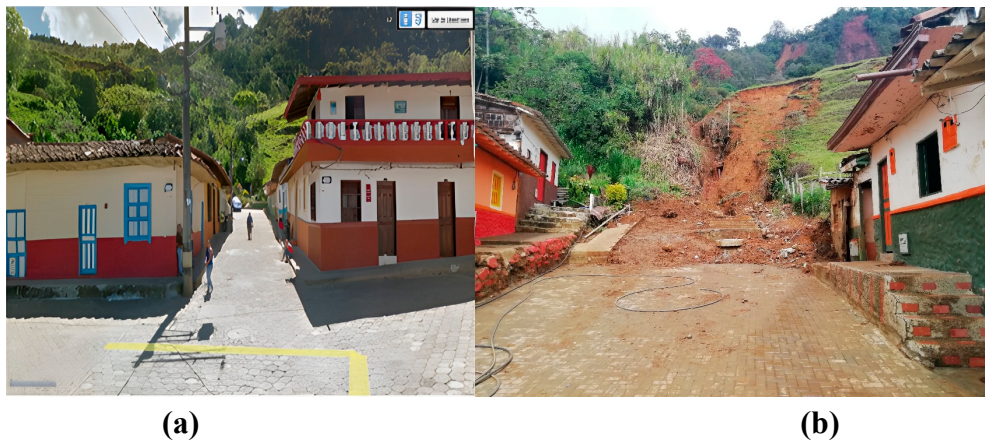
Figure 15. (a) Architectural view of houses located on 6th Street and the lower part of the slope of Las Nubes Hill. Source: Google Earth; (b) View of affected houses on the hillside of Las Nubes Hill, Valladares Stream, 6th Street. The photo was taken after evacuating the debris flow.
