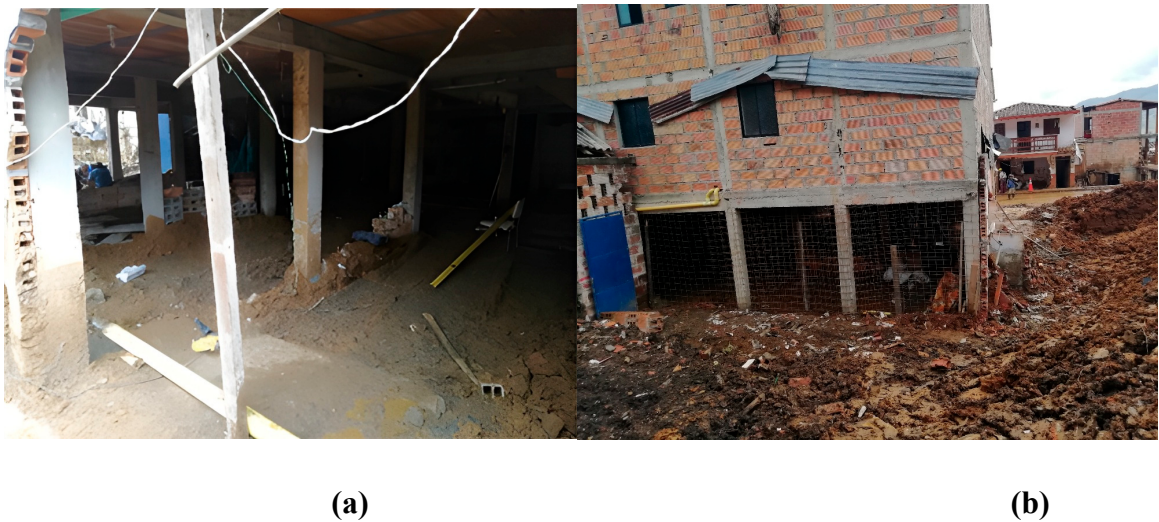
Figure 5. (a) The reinforced first storey with reinforced concrete frames. Interior view. house 2; (b) Rear facade. House 2. Reinforced with reinforced concrete wall in the first storey.
