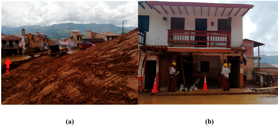
Figure 10. (a) Affected building 1 st Avenue – 7 th Street, left side. House 5; (b) The facade affected, house 5, 1 st Avenue – 7 th Street, left side.
