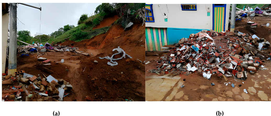
Figure 8. (a) House 4 Collapsed by the landslide; (b) Debris from House 4 due to landslide.
