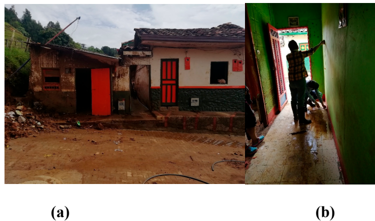
Figure 16. (a) Affected houses on the hillside of Las Nubes Hill, Valladares stream. 6th Street; (b) Debris level measurement of houses affected hillside of Las Nubes Hill, Valladares stream. 6th Street. The photo was taken after evacuating the debris flow.
