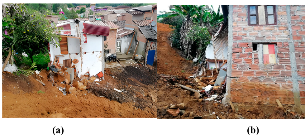
Figure 7. (a) Partially confined masonry structure. Side facade. House 3; (b) Partially confined masonry structure. Front facade. House 3.
