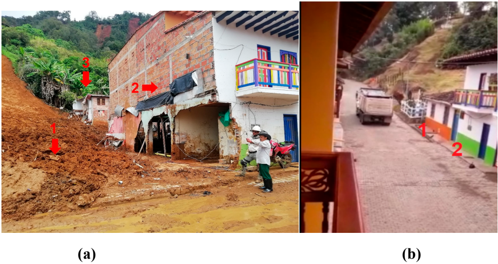
Figure 4. (a) Affected buildings. 1 st Avenue – 7 th Street, right side; (b) Buildings before the event. 1 st Avenue – 7 th Street, right side.
