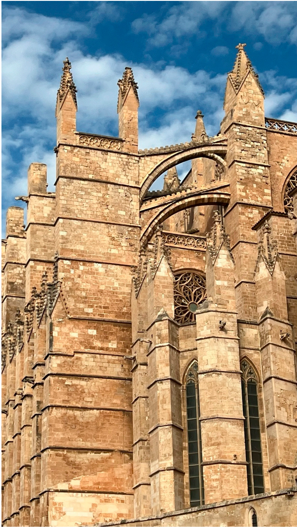
Figure 3. Exterior detail view of Palma Cathedral showing buttresses, flying buttresses, and pinnacles constructed from marés stone (photograph by the author).
