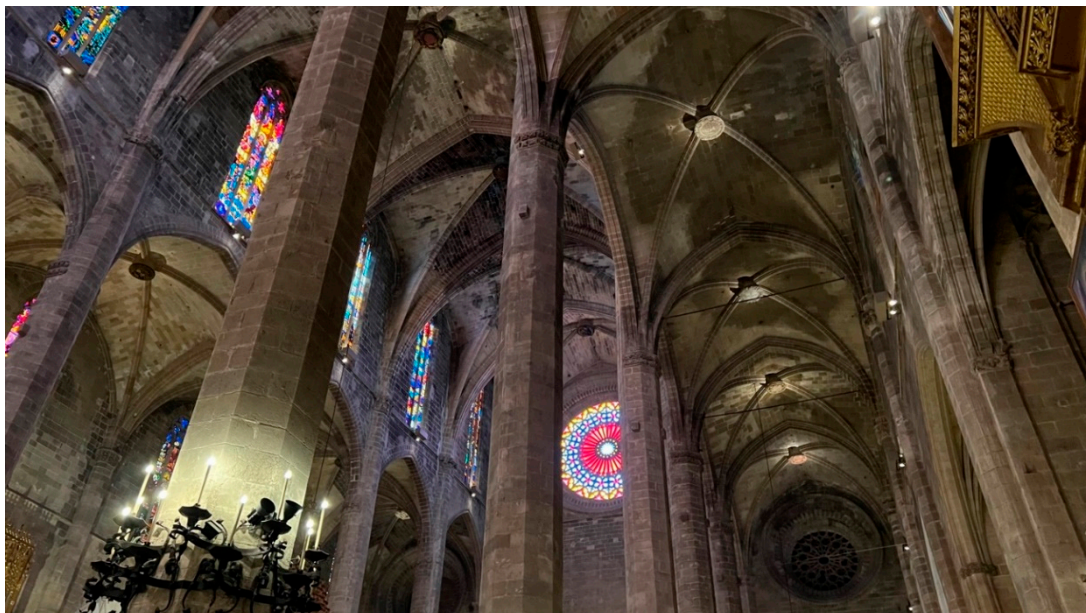
Figure 2. General interior view of Palma Cathedral, taken from one of the side aisles, showing the slender octagonal piers supporting the structure (photograph by the author).
