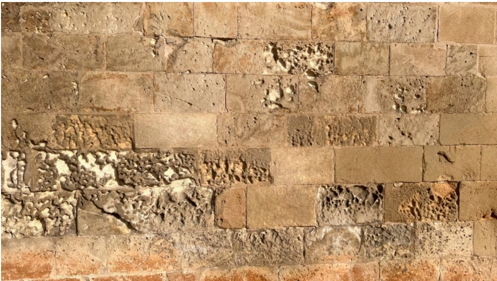
Figure 6. Wall section showing a combination of pathologies: granular disintegration, alveolization, and black crusts on the surface of mares sandstone. A restored area using a different material is also visible (photograph by the author).
