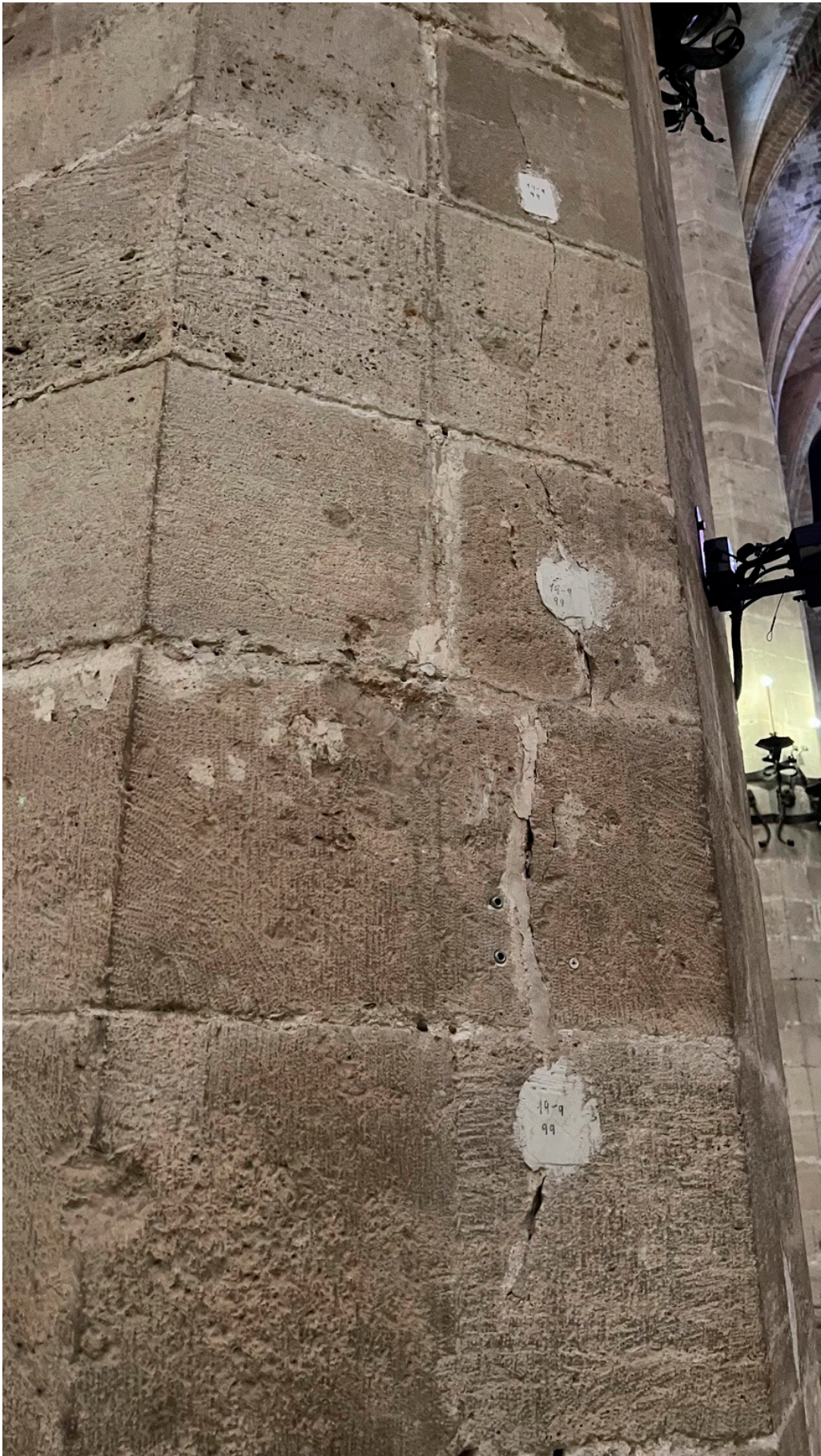
Figure 12. Cracked pier with gypsum monitoring markers (photograph by the author).
