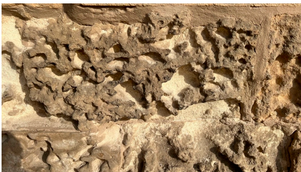
Figure 7. Advanced-stage alveolization. The loss of material volume compromises the geometry of the ashlar block (photograph by the author).
