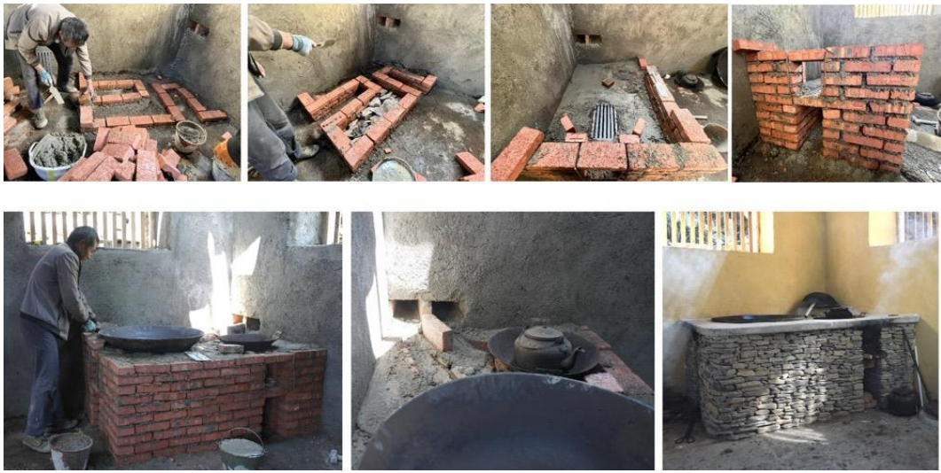
Figure 6. On-site traditional stove construction process.
