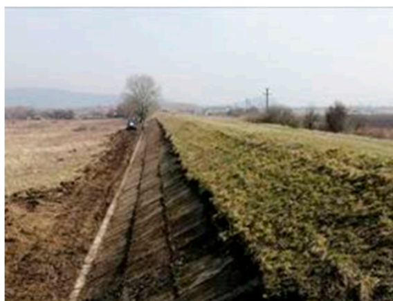
Figure 7. View of Deva flood protection levee
