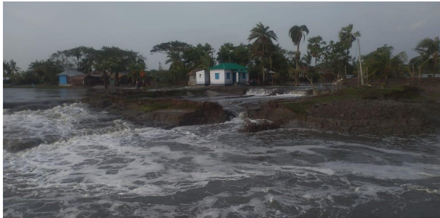
Figure 7. Part of an embankment in Shyamnagar damaged during cyclone Amphan in 2020. Source: Field data.
