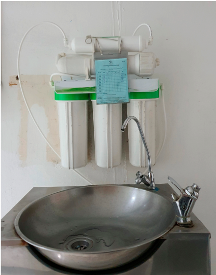
Figure A3. Commercial membrane filtration system.
