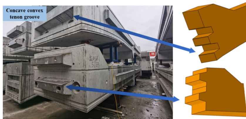
Figure 3. Concave-convex tenon groove design.
