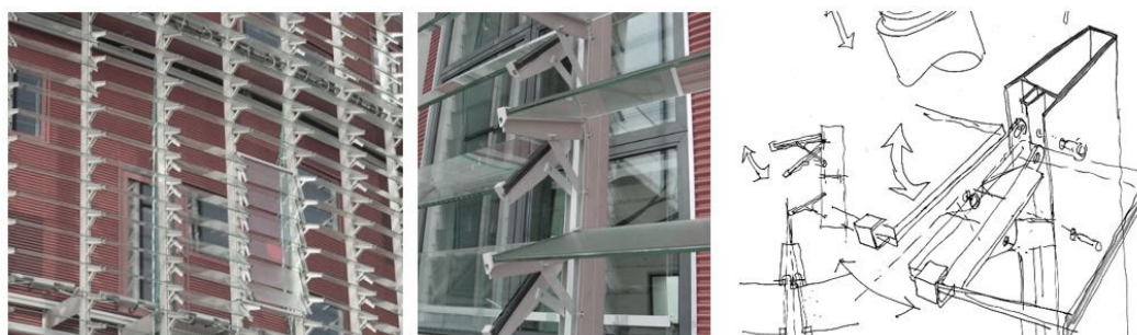
Figure 3. Agbar Tower brainwave idea; double skin façade slats fixation system.
