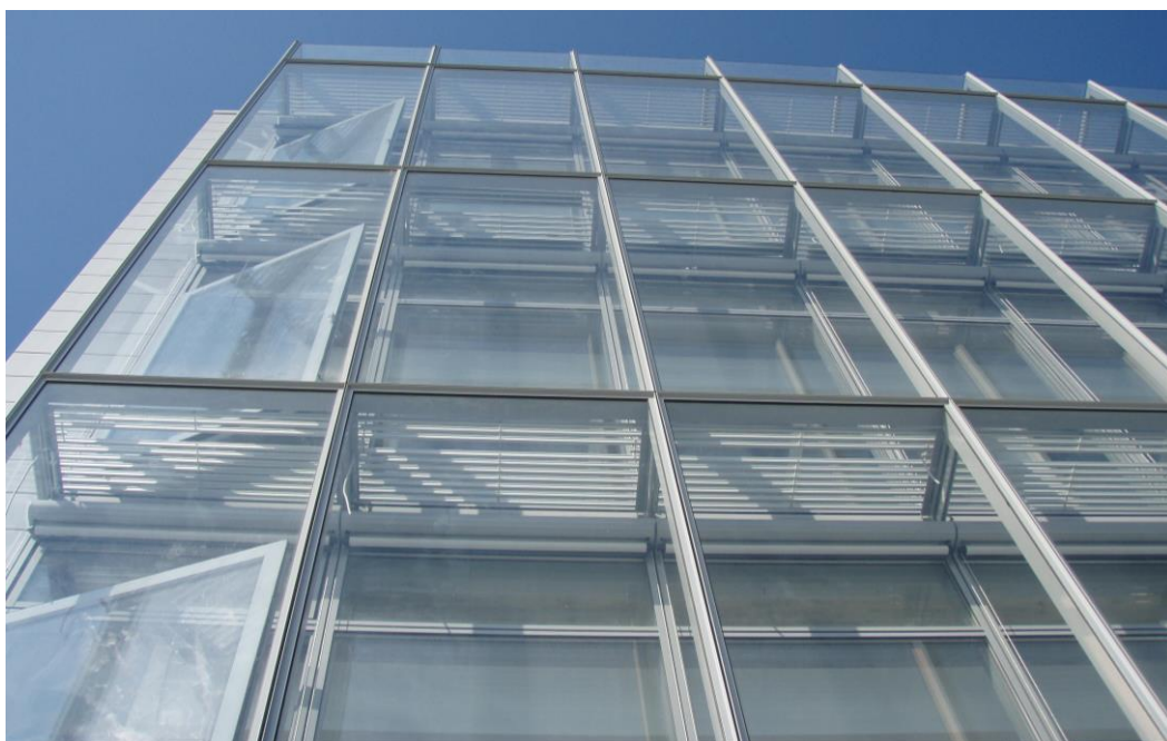
Figure 16. Sustainable methods of the multistory systems (Maurizio Varratta, iGuzzini Lab, Recanati). Composition of the envelope according to the direct gain functional procedures and cavity ventilation. Source: Pichler Projects.
