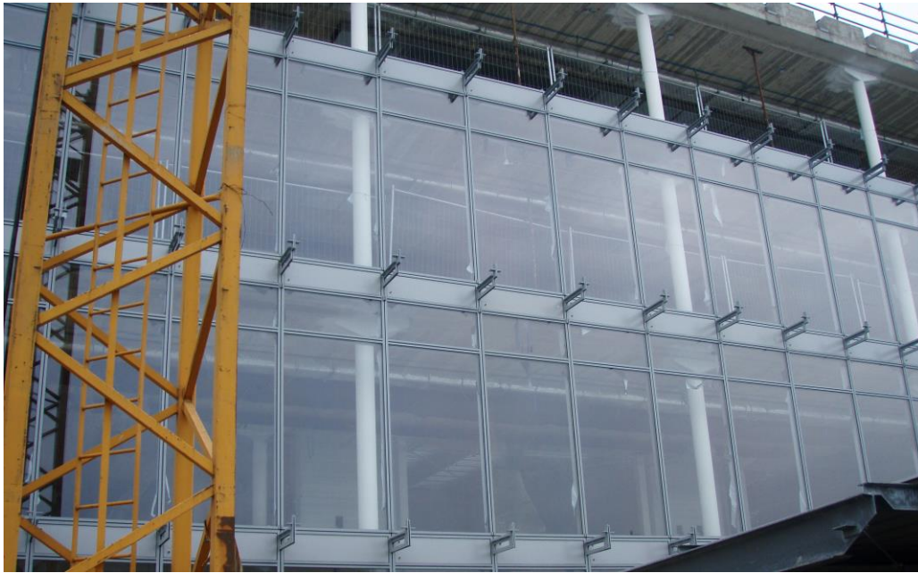
Figure 19. Sustainable methods of the multistory systems (Maurizio Varratta, iGuzzini Lab, Recanati). Construction of the curtain and brackets facing the outer screen. Source: Pichler Projects.
