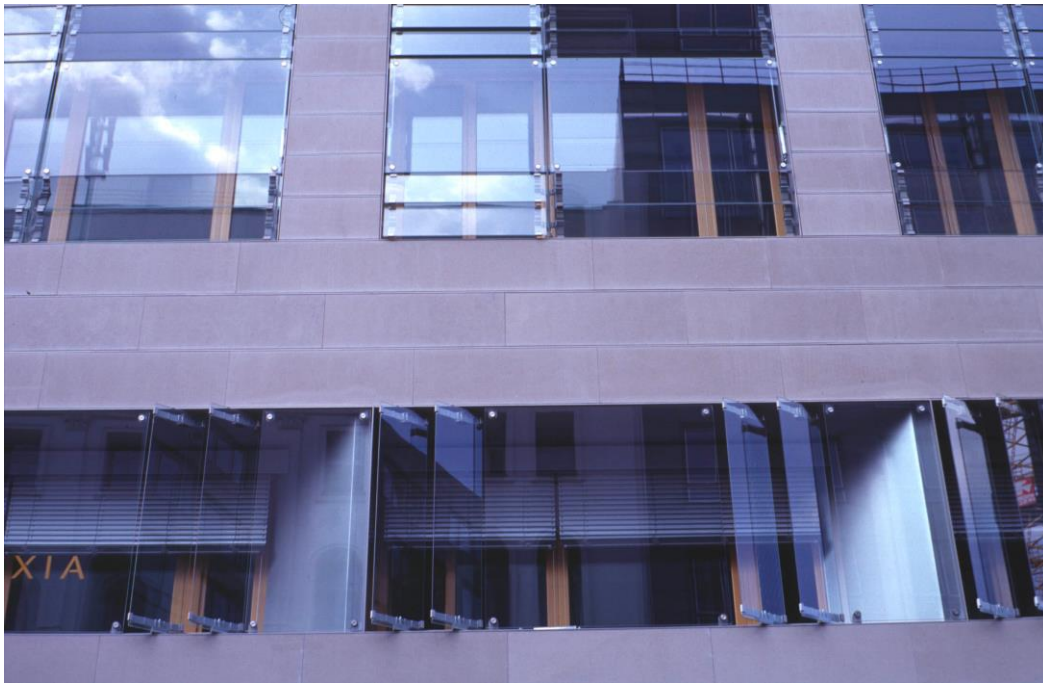
Figure 29. Application of glass screen directed to form a box-window façade. Source: Author.
