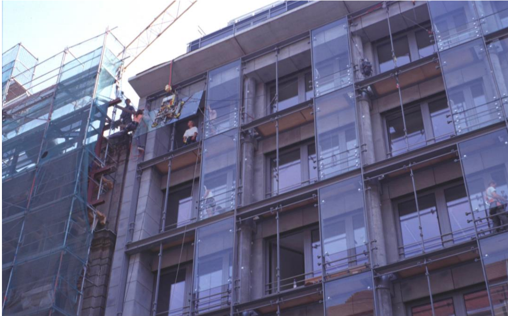
Figure 35. Application of a multistory screen made of glass modules assembled to the existing curtain using aluminium frames and mechanical fixing points. Source: Author.
