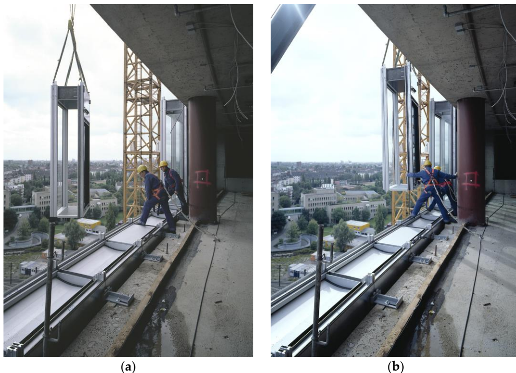
Figure 23. Sustainable methods of the multistory systems (Foster + Partners with Rhode, Kellermann and Wawrowsky, Arag Headquarter, Düsseldorf). Construction sequences: (a) The execution involves the lifting of the components by means of ropes attached to the profiles; (b) The operators engage in the slots from the brackets and the telescopic connection. Source: Gartner.
