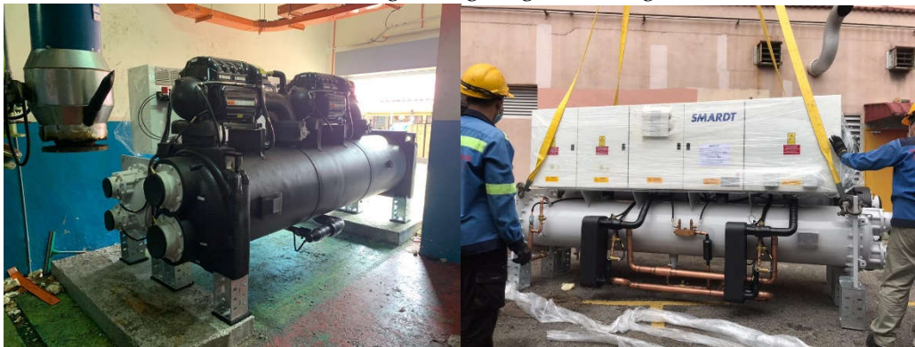
Figure 4. Oil-Free Compressor for Chiller System during Retrofit Program by Energy Performance Contracting with zero initial capital cost.
