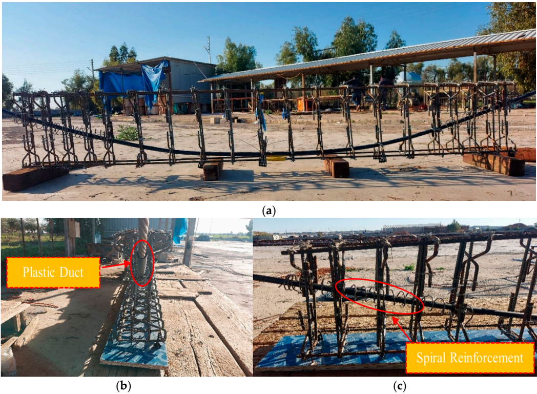
Figure 5. Reinforcement preparation: (a) Beam reinforcements detail. (b) Strand in plastic duct. (c) Spiral reinforcement.
