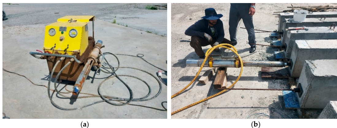
Figure 7. (a) Post-tensioning machine. (b) Applying post-tensioning force.
