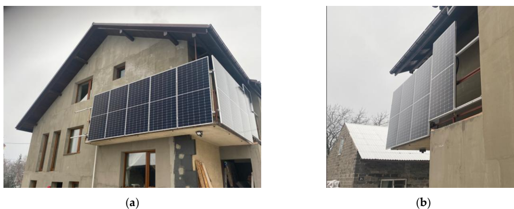
Figure 4. Balcony PV installation – detached building with roof-top with two PV fasades: (a) Southfacing and (b) East-facing (one PV module is temporarily taken off for maintenance during the photo session) in winter [Own source].
