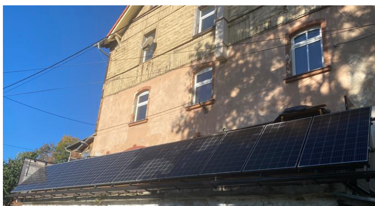
Figure 2. Case 1 - balcony PV installation – shading caused by nearby trees (only the 12 leftmost PV panels are considered, as the one rightmost operate in off-grid mode) [Own source].
