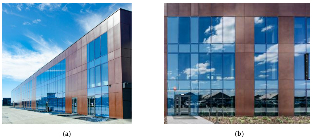
Figure 5. Façade with 22,7 kWp ventilated PV panels (the brown area) – glazed office building façade [Source: ML System S.A.; reproduced with owner permission].
