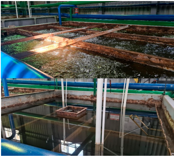
Figure 3. The second stage of aeration (above) and the site where water samples are taken from the tertiary decanting tank (below).
