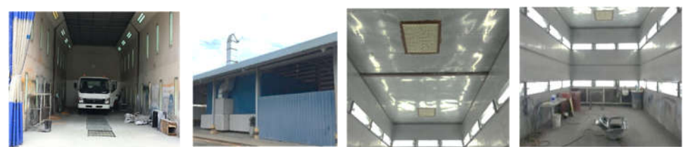
Figure 3.3. Designated spray paint area with an Local Exhaust Ventilation System(LEV).
