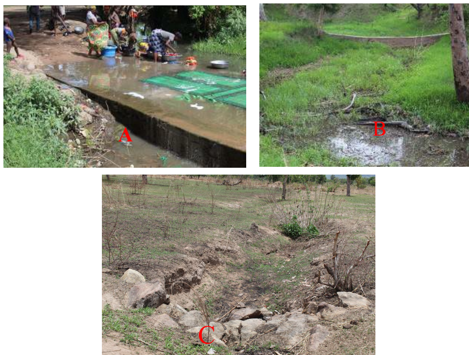
Plate 1. Masonry (A and B) in Ndock and stone wedged " biefs " (C) in Sabongari. (Source: Tchuenga, March 2022).
