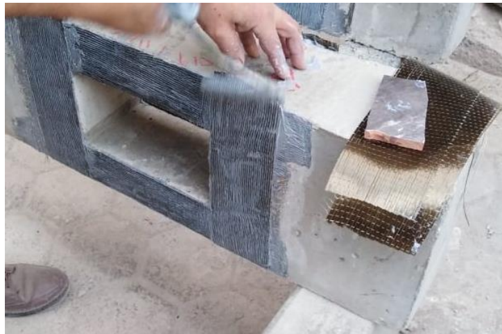
Figure 8. Installing of the BFRP Sheet.
