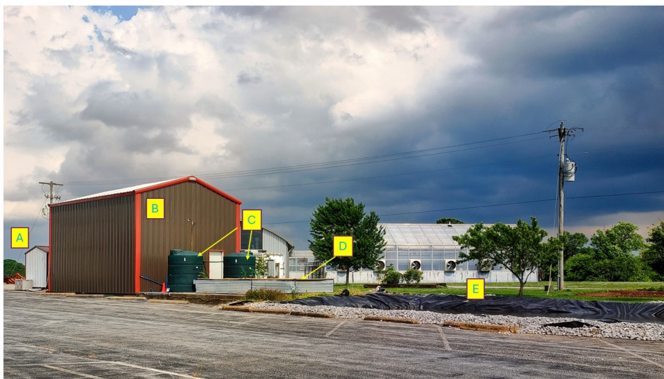
Figure 1. Anaerobic Digester/Wastewater treatment complex. A. Shed containing audio amplifiers and recording equipment. B. Building housing feeding tank, anaerobic digester, aeration tank, C. Holding tanks for digester effluent. D. Constructed wetland. E. Water retention lagoon for recycling back to the waste digester. Note that building houses two anaerobic digesters but that only one is fully functional at the time of this writing.
