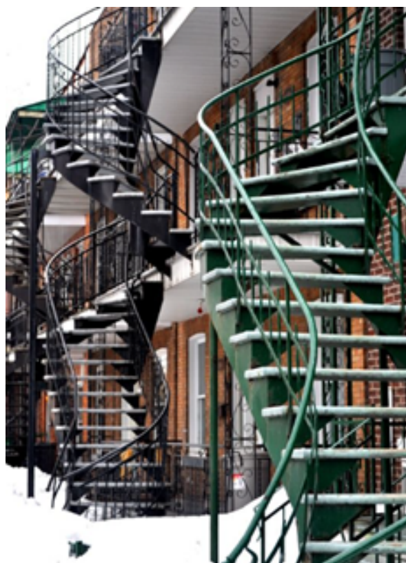
Figure 3. Montreal External Staircases (in winter).
