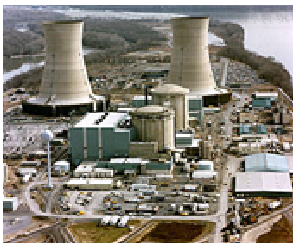
Figure 4. View of former Three Mile Island Nuclear Generating Station NPP along the Susquehanna River near Harrisburg, Pennsylvania.
