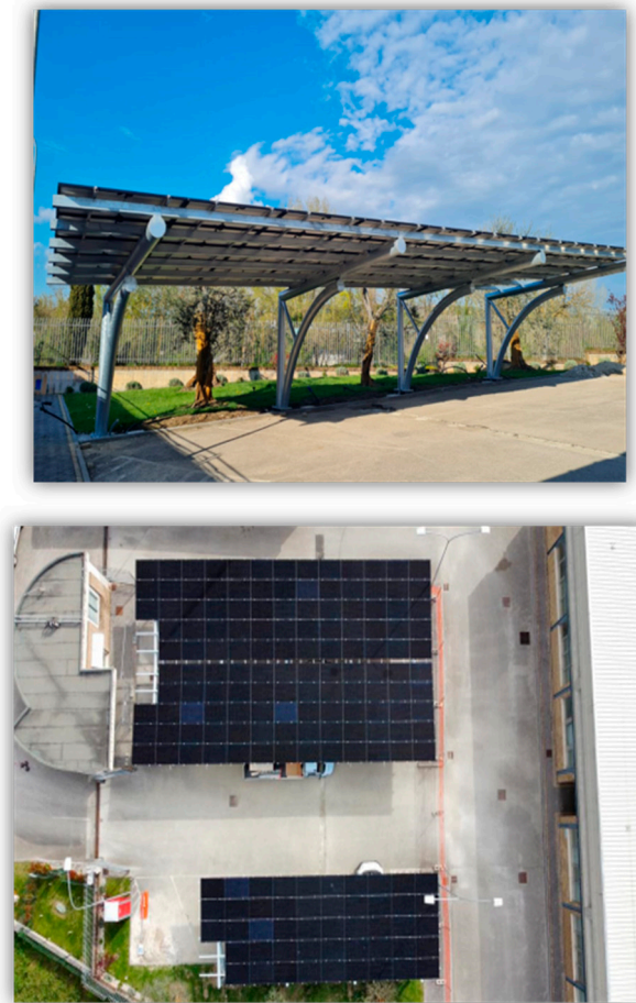
Figure 6. Finished canopies with the photovoltaic system.
