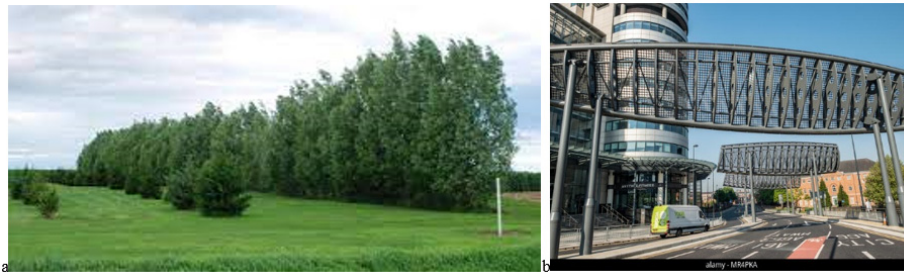
Figure 4. a. Green barriers at different heights; b. Deflectors made of steel frames covered with perforated aluminium to reduce wind speed, Bridgewater Place, Leeds, England, 2005.
