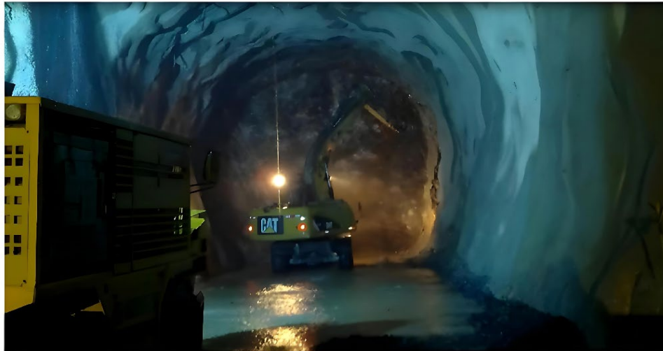
Figure 12. Excavator Operation and commissioning in the hydraulic tunnel.
