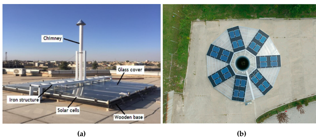
Figure 12. Utilization of photovoltaic panels in solar chimneys: (a) Utilizing solar panels inside the collector [96], (b) Utilizing solar panels on the collector, with visible components such as the central chimney, surrounding glass collector area, and symmetrically arranged rectangular solar panels on each collector segment, reproduced with permission No. 5937220512580 [97]
