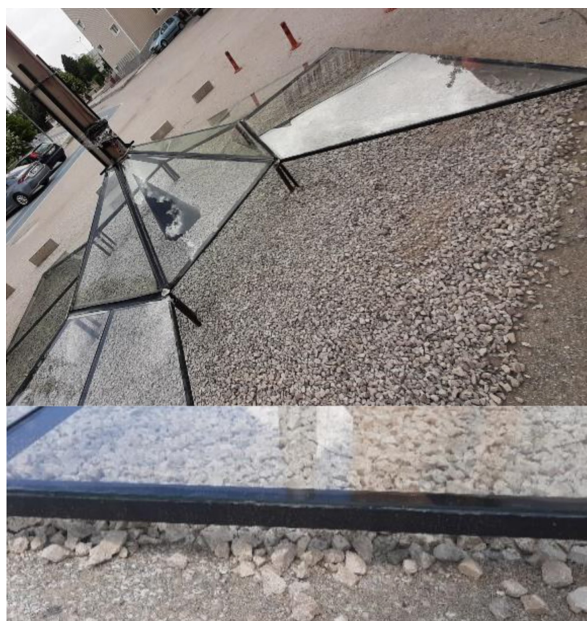
Figure 11. Use of crushed gravel inside the collector, reproduced with permission No. 5937210444412 [73]
