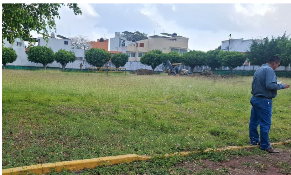
Figure 2. Reactivating disused wells. Town hall staff overseeing work that has begun on a disused oil well in the Cazonos neighbourhood, Poza Rica, Veracruz. Source: Authors.
