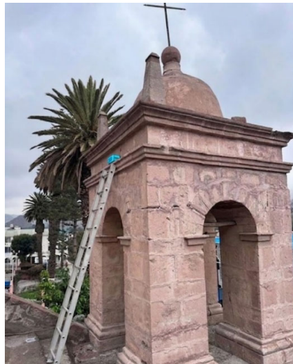
Figure 2. Ambient vibration measurements using a TROMINO® seismograph at different locations of the church (tower and roof).
