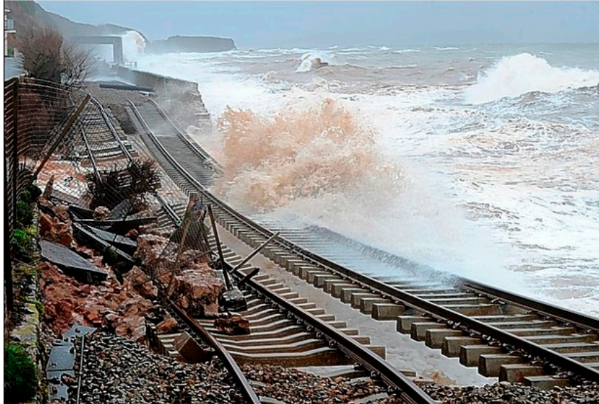
Figure 16. The main railway line to Cornwall and Devon was demolished at Dawlish by storms which hit the UK in February 2014 [41-42].
