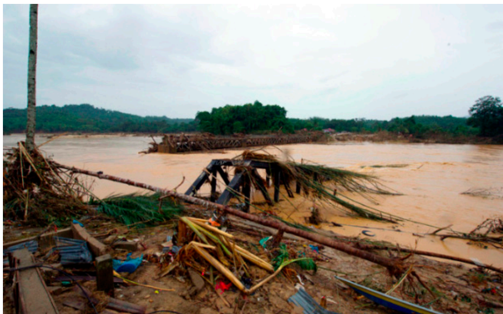
Figure 5. Malaysia East Coast Line railway bridge which cross Nenggiri River in Kemubu, Kelantan had totally lost due to massive flood in December 2014 (courtesy: Malaysia Department of Public Works).
