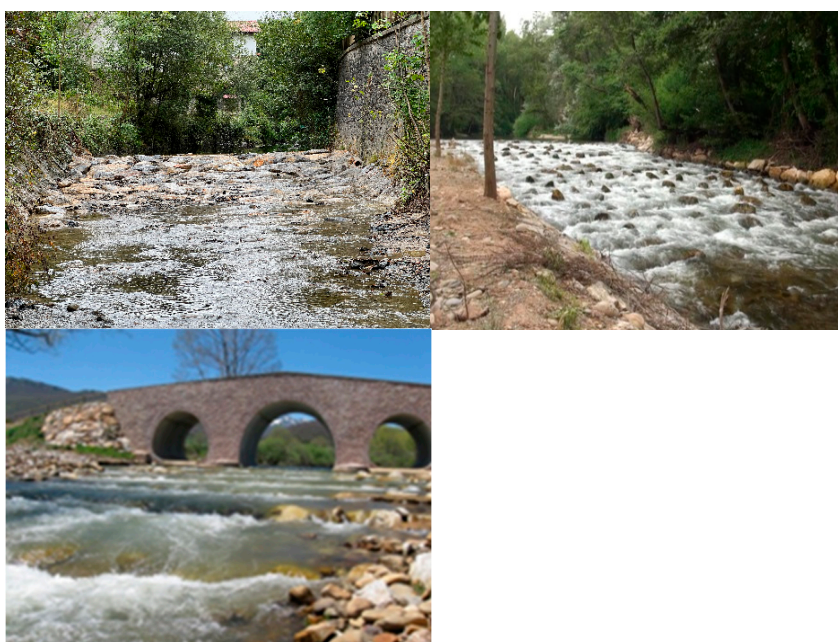
Figure 2. Left: bottom semi-dry ramp in Azkoitia (Gipuzkoa). Center: boulder ramp [R-bl-c] in the Najerilla River, La Rioja). Right: concrete pool-and-weir ramp [R-pw-c] in the Pisuerga River, northern Palencia.
