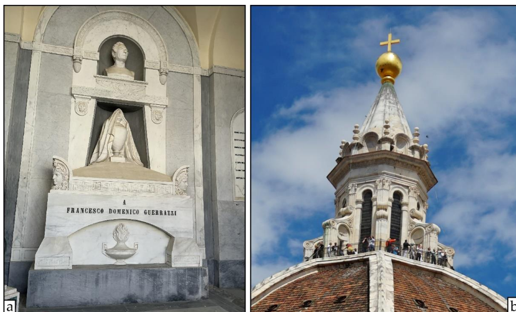
Figure 10. Examples of some monuments made with CMM. (a) Tomb of Francesco Domenico Guerrazzi at the cemetery of Montenero, Livorno. (b) The Lanterna of the Brunelleschi's Dome of the Santa Maria del Fiore Cathedral in Florence; the top cone is made up with CMM. (Phots by G. Risaliti and M. Coli)
