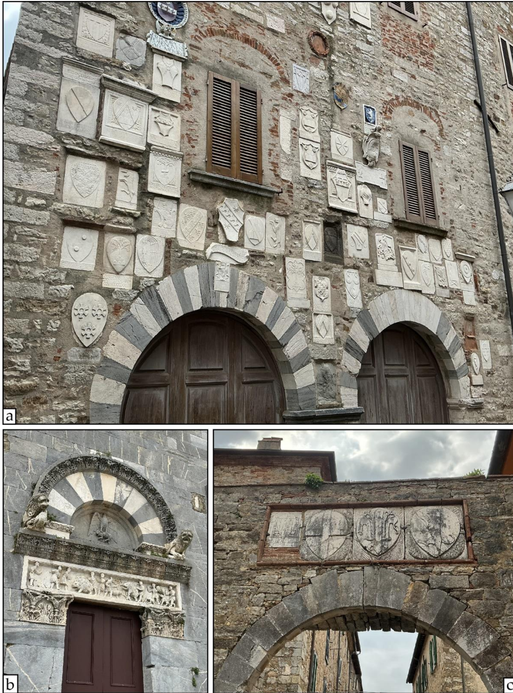
Figure 2. Examples of some buildings in Campiglia Marittima where CMM were used as quoins, ashlars or coats of arms. (a) Palazzo Pretorio; (b) external door of the parish church of San Giovanni; (c) North gate of the city walls. (Photos by G. Risaliti).
