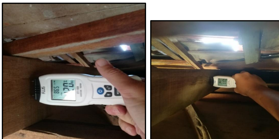
Figure 3. Moisture Contents Inspection.
