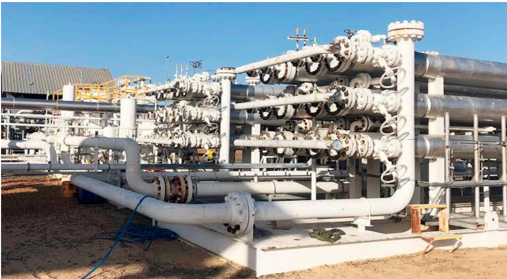
Figure 9. Gas separation Membrane for CO 2 Removal.
