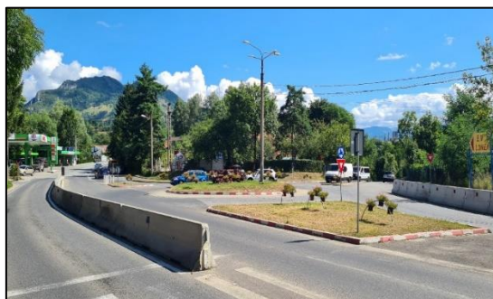
Figure 35. Daranesti roundabout – intersection edge.
