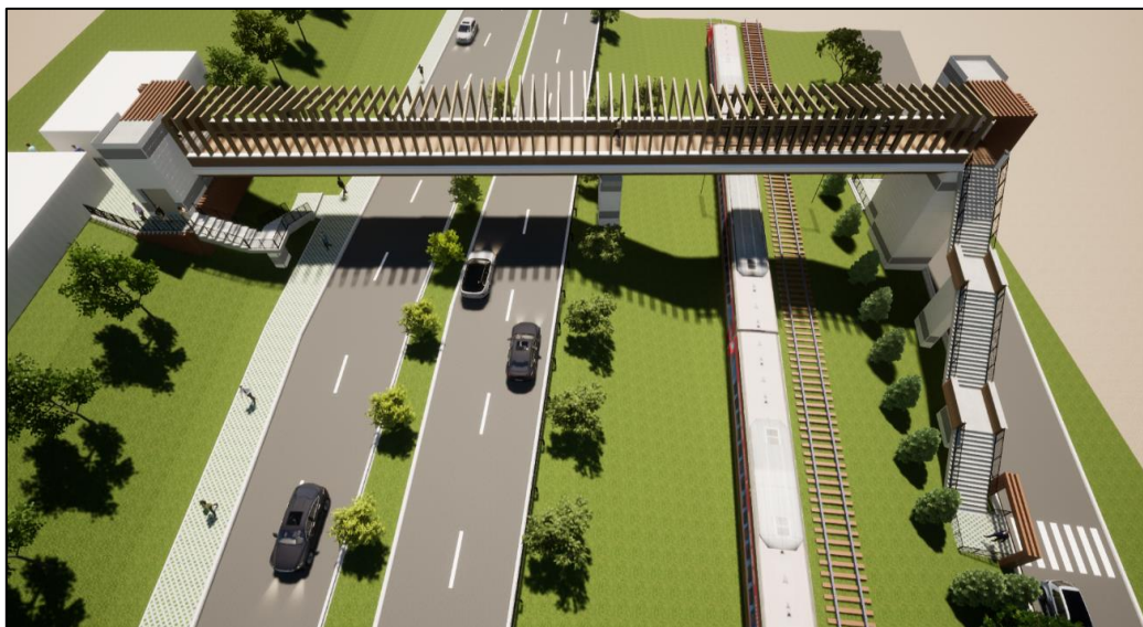
Figure 141. Footbridge 1 - Lunca area (source: S.C. VENTOR Grup Consulting S.R.L.).
