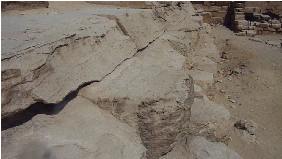
Figure 30. Wear or erosion of the paving immediately outside the cladding blocks at point 15.
