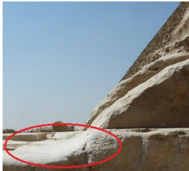
Figure 15. Wear on the paving immediately outside the paving blocks at point 6, highlighted in the red oval.
