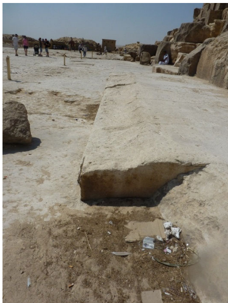
Figure 17 and 18. Wear or erosion of the paving immediately outside the cladding blocks at point 7.
