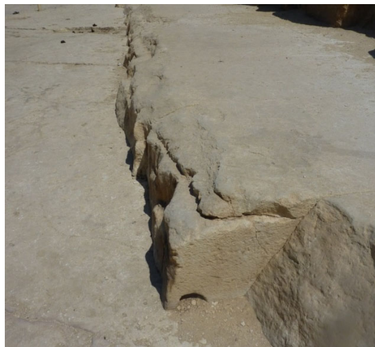
Figure 22. Wear or erosion of the paving immediately outside the cladding blocks at point 11.
