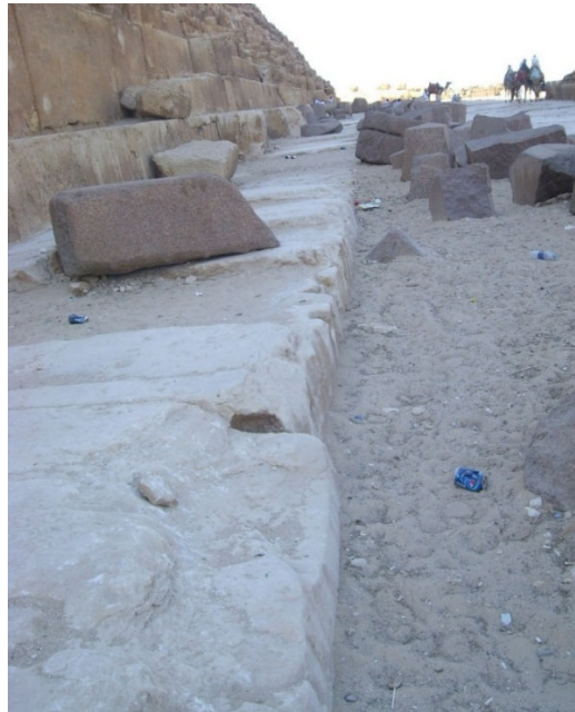
Figure 34. Wear or erosion of the paving immediately outside the cladding blocks at point 18.
