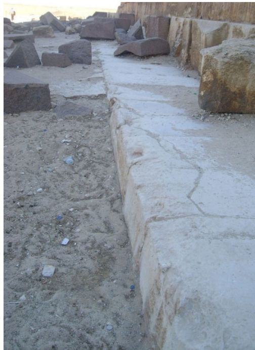
Figure 35. Wear or erosion of the paving immediately outside the cladding blocks at point 19.
