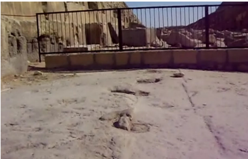
Figure 43. Wear or erosion of the pavement immediately outside the paving blocks at point 25.
