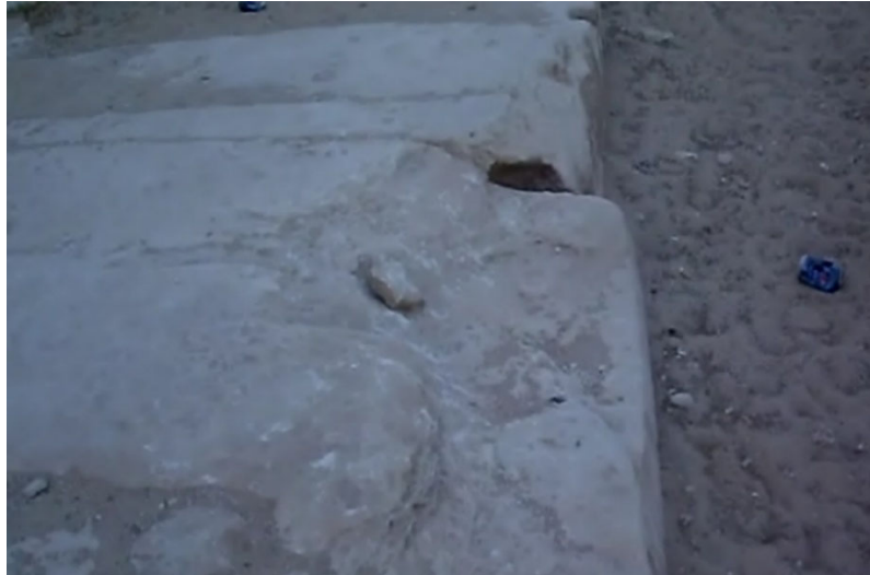
Figure 36. Wear or erosion of the paving immediately outside the paving blocks at point 20.
