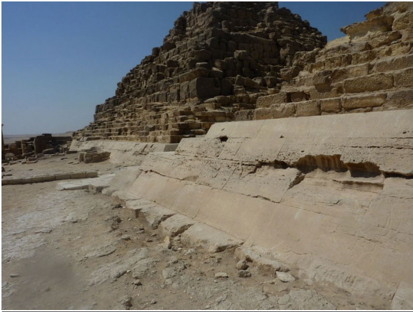
Figure 28. Wear or erosion of the paving immediately outside the cladding blocks at point 14.
