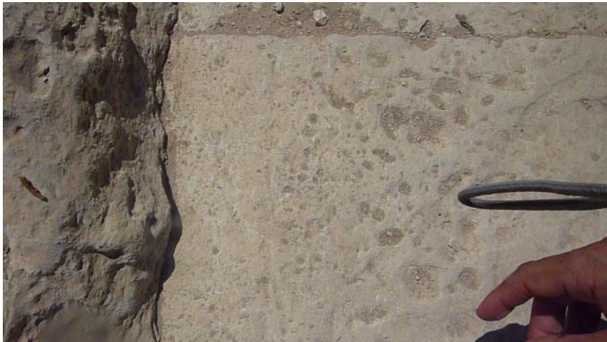
Figure 23. The difference in erosion at point 12 between the right side (which has been exposed since the pyramid was built) and the left side.
