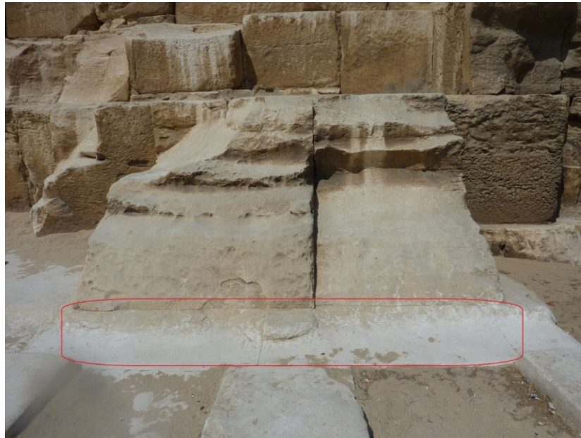
Figure 16. Wear on the paving immediately outside the cladding blocks at point 6, highlighted in the red rectangle.
