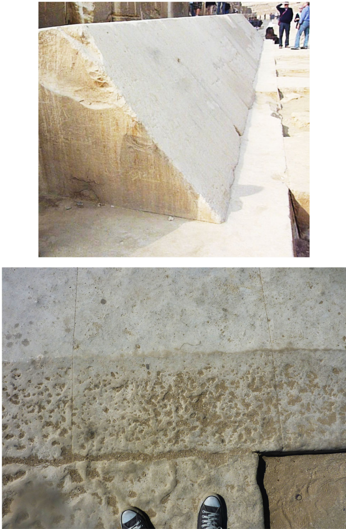
Figure 8 and 9. Detail of the Pyramid of Khufu at point 1. On the left are the only remaining limestone cladding blocks, and on the right is the clear difference in erosion between the lower part (which has been exposed since the pyramid was built) and the upper part (which has only been exposed to erosive agents for 675 years).
