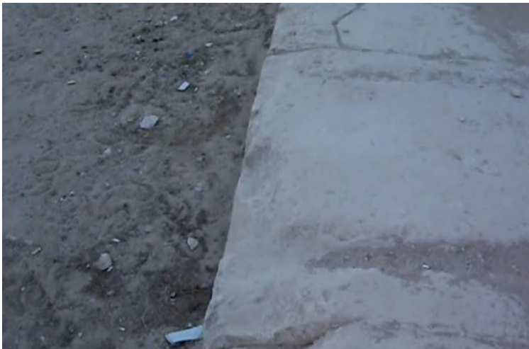
Figure 38. Wear or erosion of the paving immediately outside the cladding blocks at point 22.
