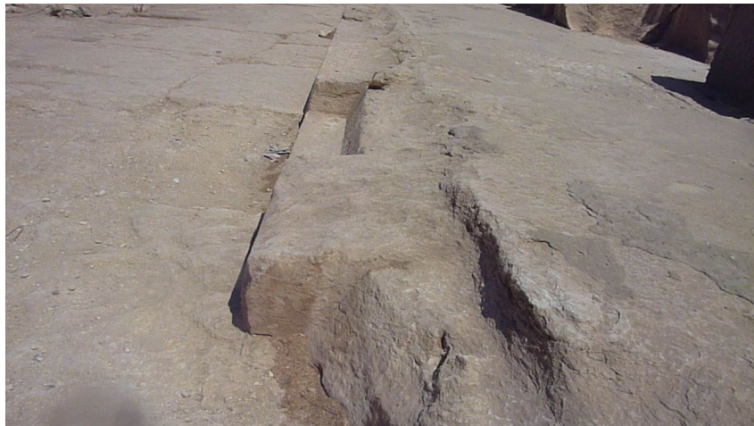
Figure 20. Wear or erosion of the paving immediately outside the cladding blocks at point 9.
