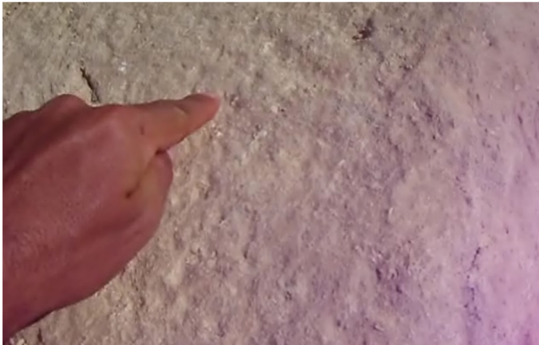
Figure 42. Erosion of the base of the pyramid of Khafra carved into the rock, which was once covered by cladding blocks, at point 24.
