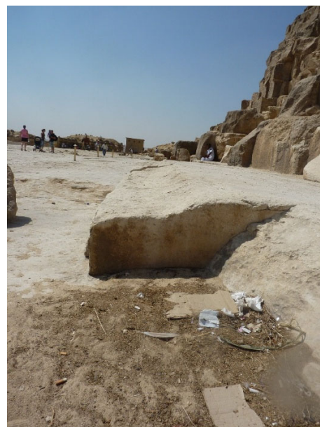
Figure 17 and 18. Wear or erosion of the paving immediately outside the cladding blocks at point 7.
