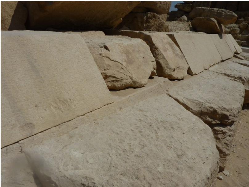
Figure 31. Wear or erosion of the paving immediately outside the cladding blocks at point 16.
