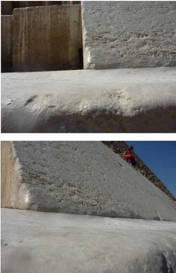
Figure 12 and 13. Wear of the paving immediately outside the cladding blocks at point 3.
