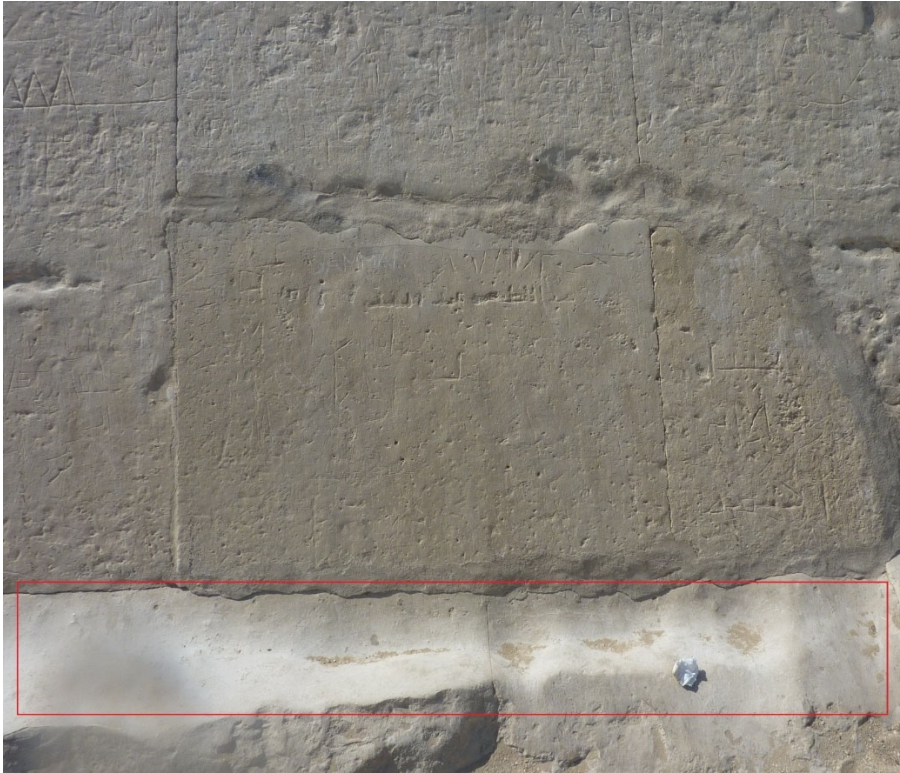
Figure 14. Wear on the paving immediately outside the cladding blocks in point 3, highlighted in the red rectangle.
