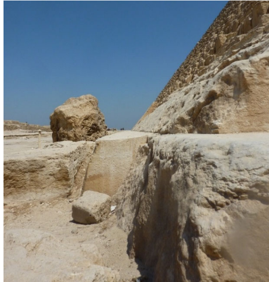
Figure 21. Wear or erosion of the paving immediately outside the cladding blocks at point 10.
