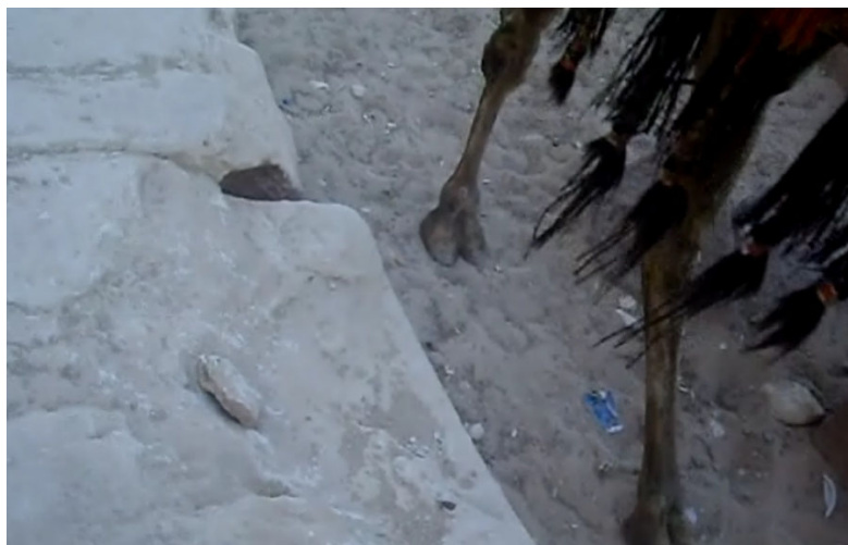
Figure 37. Wear or erosion of the paving immediately outside the cladding blocks at point 21.
