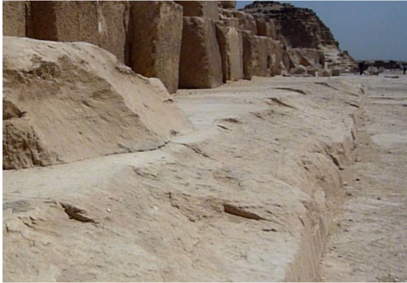
Figure 19. Wear or erosion of the paving immediately outside the cladding blocks at point 8.
