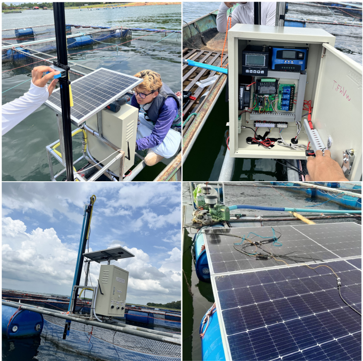
Figure 9. Installing water quality control nodes.
