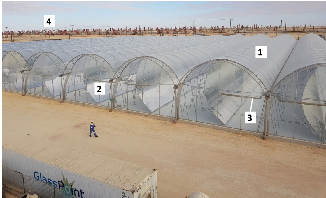
Figure 8. An aerial view of the Amal II pilot project (© GlassPoint, reproduced with permission). (1) Protective greenhouse enclosure, (2) Parabolic trough collector mirror, (3) Receiver pipe, (4) Beam pumps (pump jacks) within the oil field.
