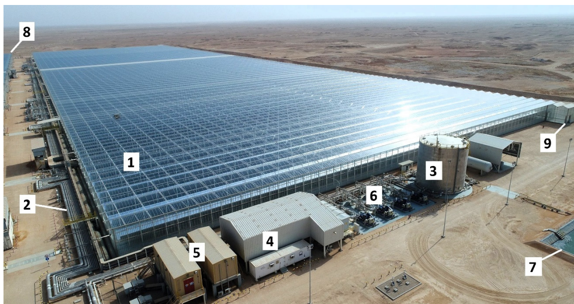
Figure 11. An aerial photo of one of the six zones of the Miraah commercial project (© GlassPoint, reproduced with permission). (1) Solar collector field (one of the six enclosures), (2) Steam distribution pipes, (3) Water storage tank, (4) Steam generation plant, (5) Control rooms/offices, (6) Pump skid (to pressurize liquid water and deliver it from the storage tank to the receiver tubes), (7) Water reservoir, (8) Adjacent solar collector enclosure.
