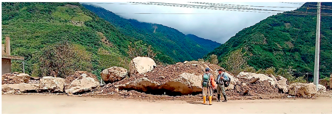
Figure 12. Panoramic view of several boulders on the E-30 road. The big one has a diameter of more than 9 m (June, 2024 event).
