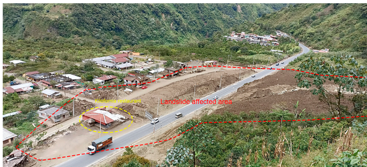
Figure C3. Details of the area affected by the mudslide. Note that the accumulation of material is located west of the restaurant.
