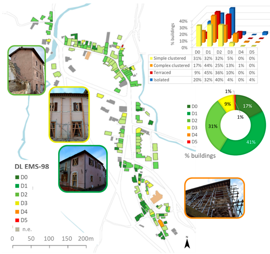
Figure 5. Distribution of damage level (DL) in buildings of Pievebovigliana according to EMS-98: map with example of damage (from D1 to D4 in pictures) and diagram of overall relative frequency; histogram of relative frequency of DL related to aggregation type of buildings.
