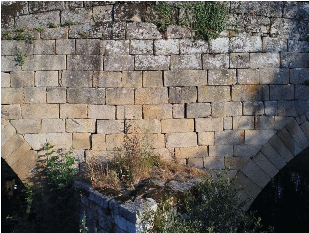
Figure 12. View of the central area of the spandrel wall, upstream of the bridge just above the starling, where the separation between some ashlars can be seen, in an image captured with the drone (photograph by the author).
