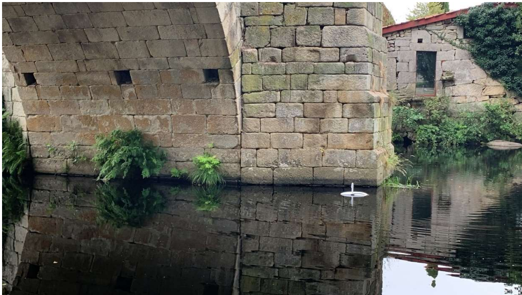
Figure 8. Underwater drone surrounding the central pier of the Vilanova Bridge from downstream/the west, inspecting the river bottom around the cutwater (photo by the author).
