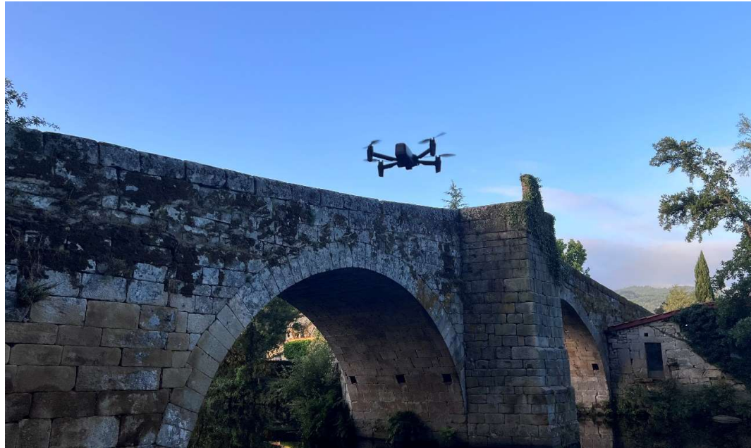
Figure 5. General view of the quadcopter drone with a thermal imaging camera used during the inspection, approaching the Vilanova Bridge for reconnaissance (photograph by the author).
