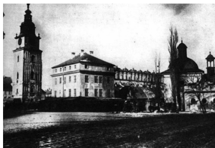
Figure 5. Historical photograph of the Great Weigh House, as seen from Grodzka Street, with Town Hall Tower (left) and St. Adalbert (right) [54].
