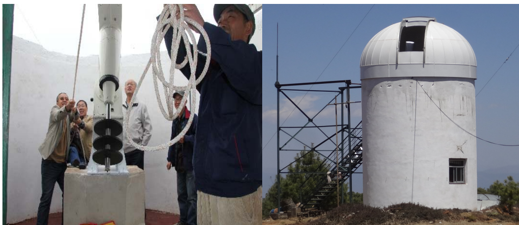
Figure 3. Light: In the early stages of YOGIS construction in 2013, the coronagraph lacked rainproof facilities. A movable rain shelter was installed on the roof of the circular building. The image shows staff members opening the roof shelter via pulleys to conduct observations. Right: In 2014, a dome was designed and installed according to the dimensions of the circular building, upgrading the equipment for safeguarding the observation environment.
