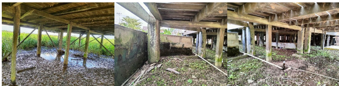
Figure 8. Foundation Condition with Dry Areas.
