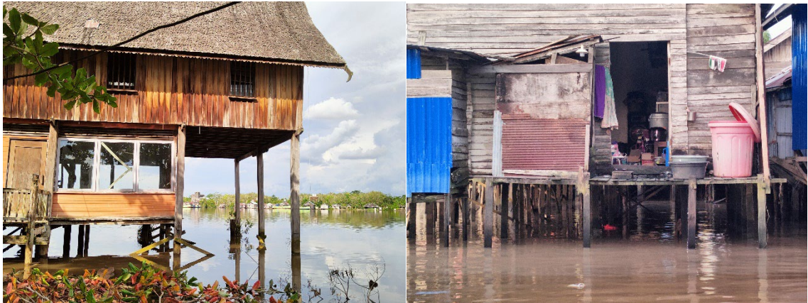
Figure 4. Foundations in Waterlogged Areas (River).
