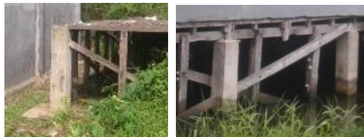
Figure 1. Combination of Wooden and Concrete Pile Foundations.
