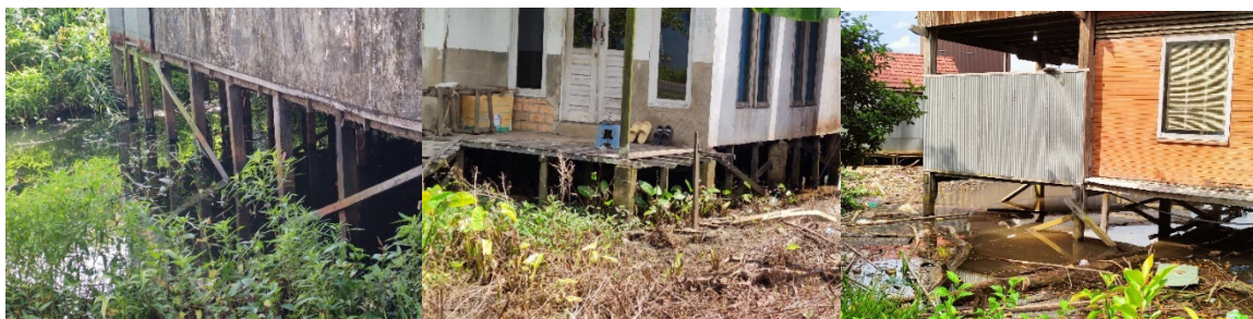
Figure 3. Foundations in swampland.
