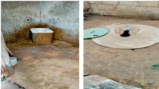
Figure 13. "Turkish" toilet and latrine with concrete lid. Source: CMM [33].
