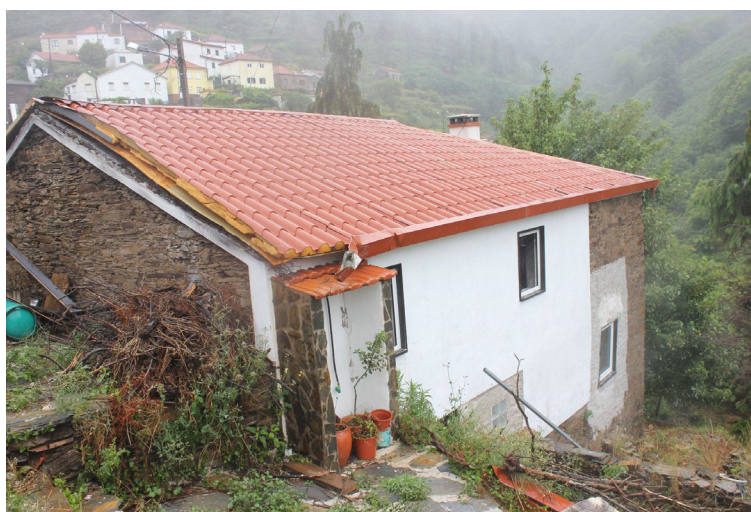
Figure 2. Location where the gas cylinders were removed.
