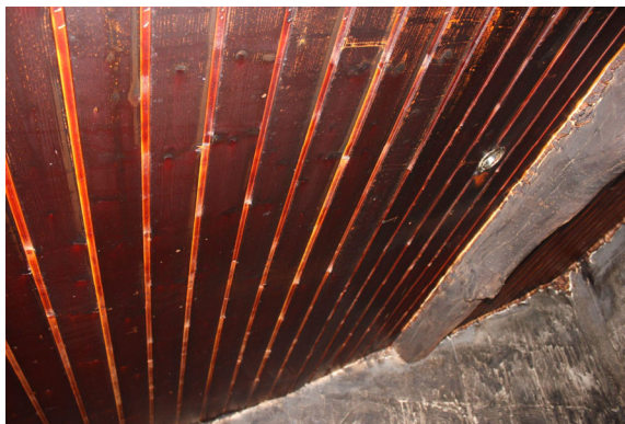
Figure 5. Location of the house where the ceiling was not consumed by fire.
