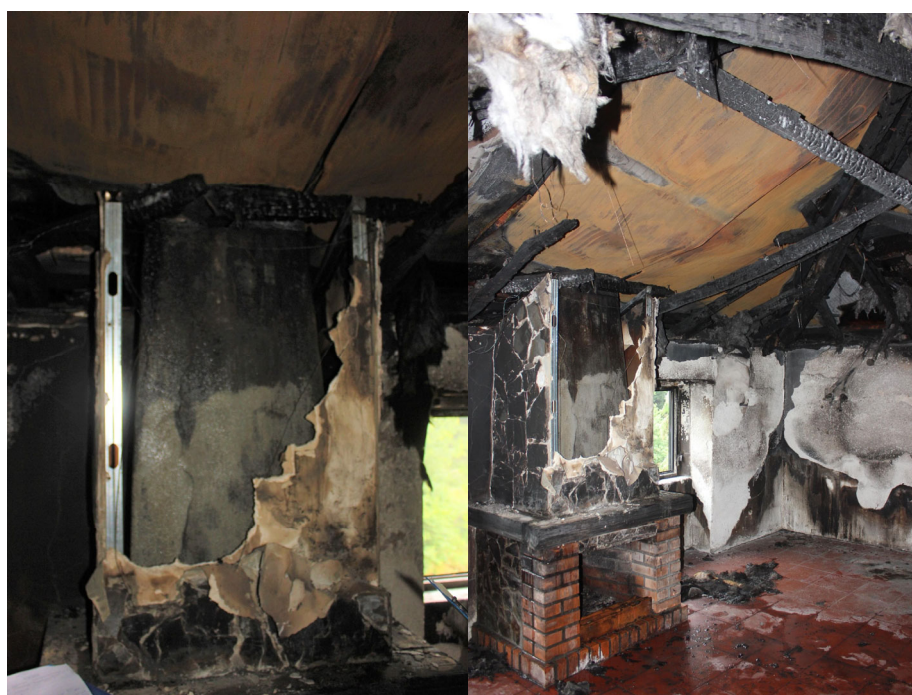
Figure 3. plasterboard wall, covered with stone, and a wooden ceiling encompassing a beam inside the fireplace, without ventilation.
