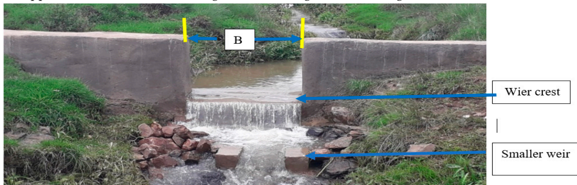
Figure 3. Stream flow measuring weir at the outlet of the research sites.
