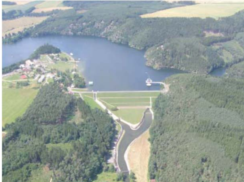
Figure 2. Water Reservoir / authors/.
